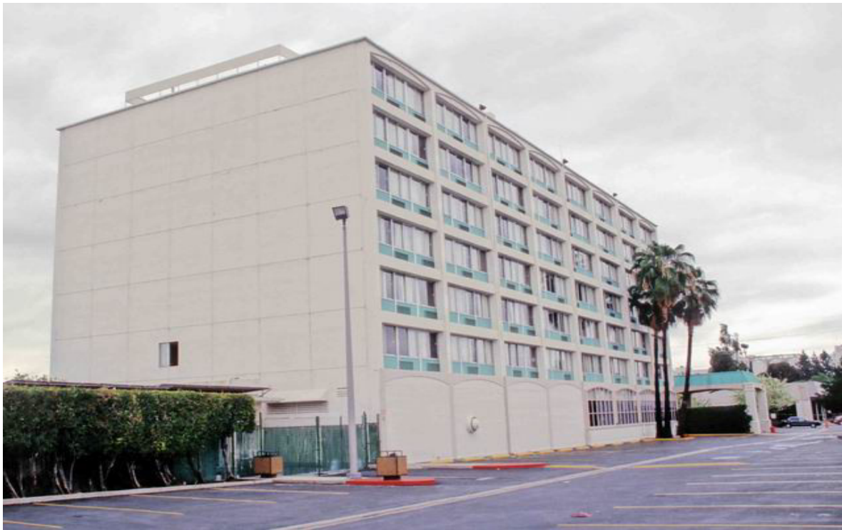
Fig. 1. View of Van Nuys Seven Story Hotel (VN7SH) from North-East.
