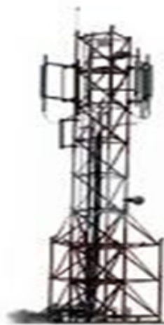
Figure 1. Picture Of Telecom Mast/Based station
